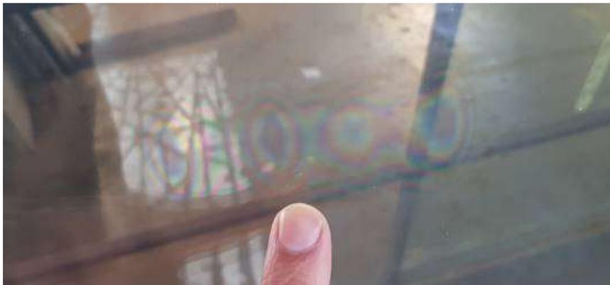
We recommend to eliminate the newton rings that are present is to remove some of the black secondary sealant to expose the SIG spacer. (See pictures below)
