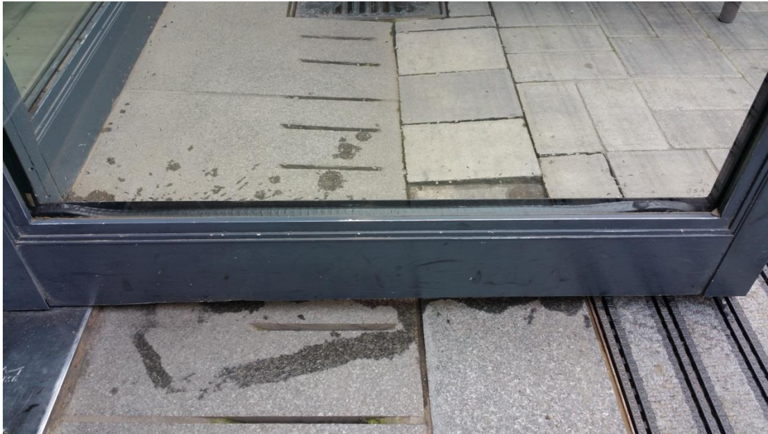
Figure 2 : Setting blocks not supporting glass, therefore units hermetic seal compromised.
