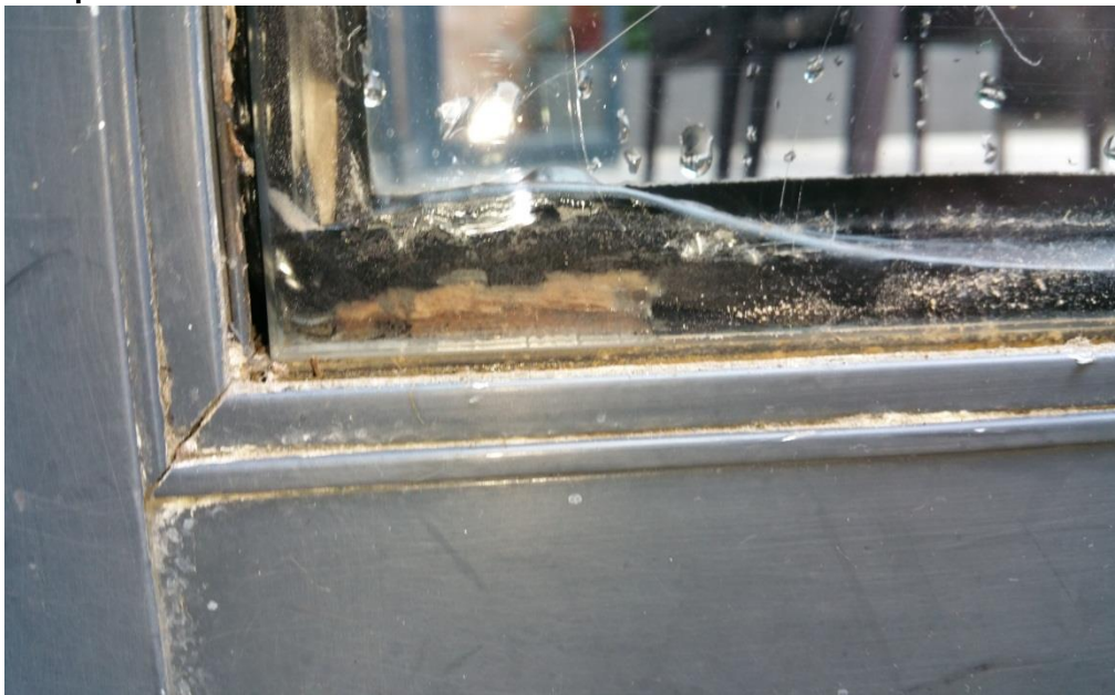
Figure 2 : Setting blocks not supporting glass, therefore units hermetic seal compromised.
